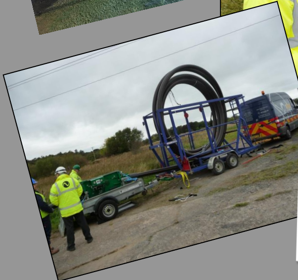
Effluent Line Slip Lining Project
