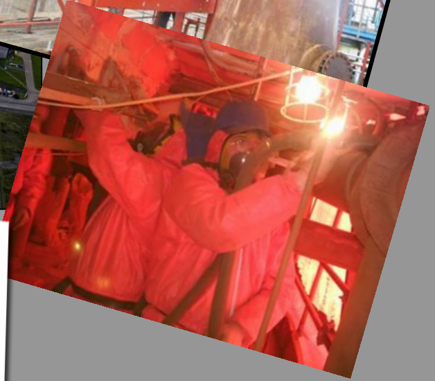
Bulk Asbestos Removal
