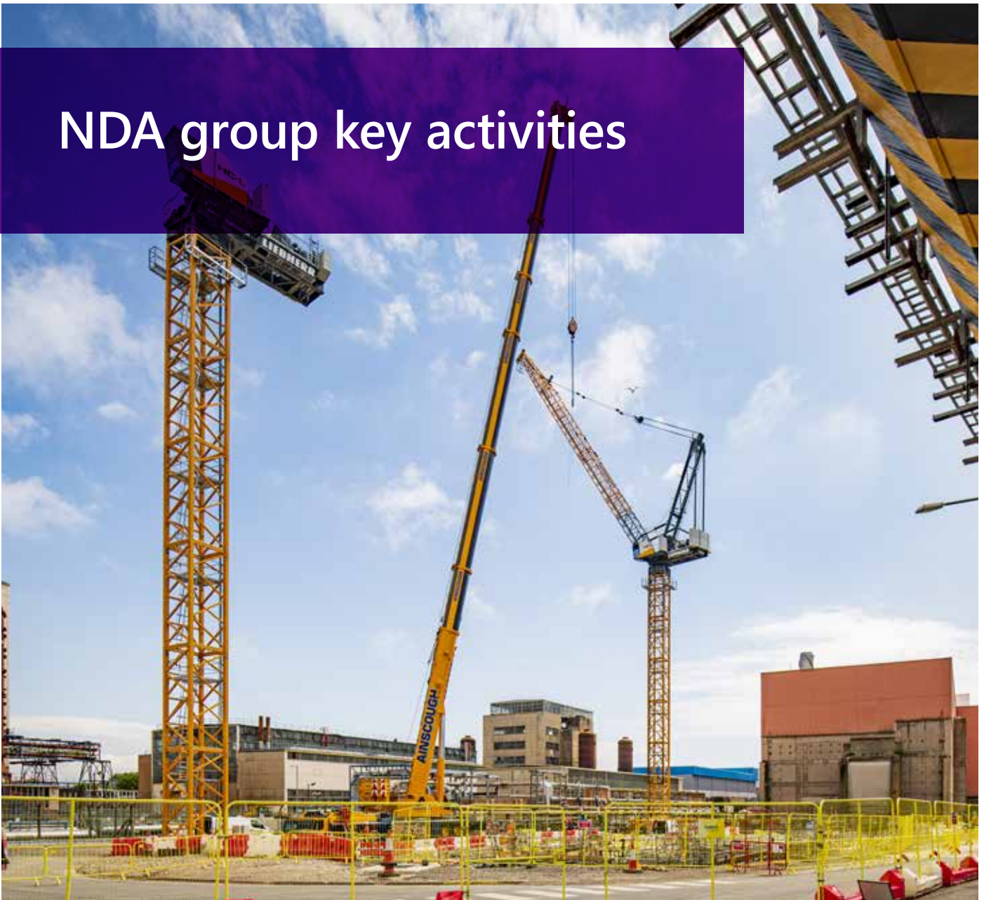
Site Ion Exchange Effluent Plant (SIXEP) Continuity Plant (SCP)
