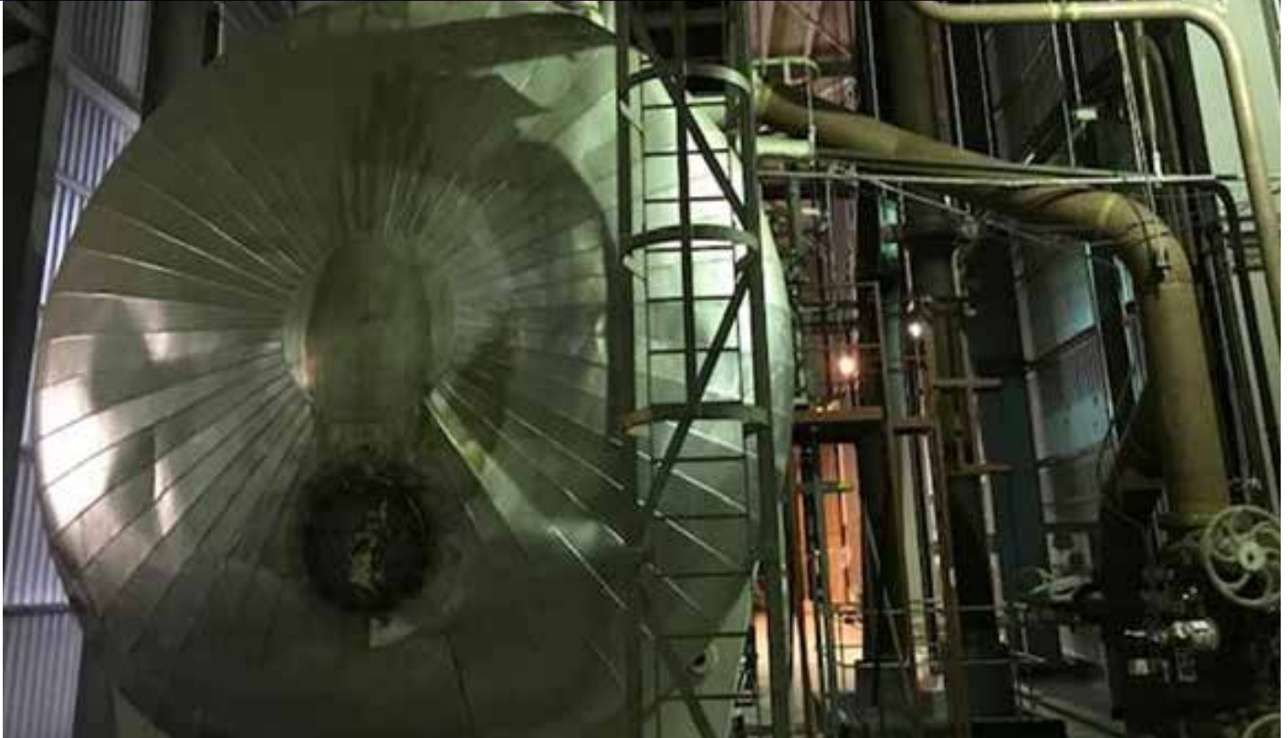
Asbestos removal at Wylfa
