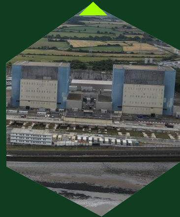
Hinkley Point A Vaults
