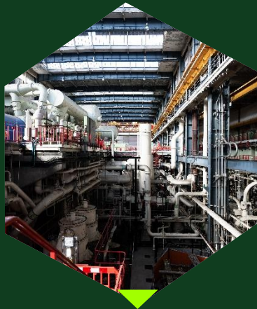
Oldbury turbine hall demolition
